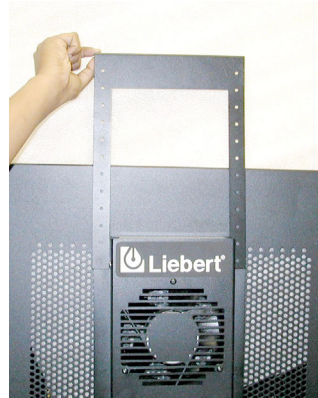
Lifting mounting bracket off XDA
